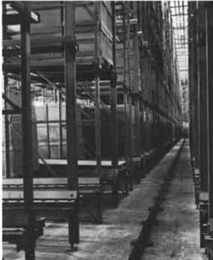
*A live storage Palletflo similar to several Navy installations for first-in, first-out handling of pallet loads.*
