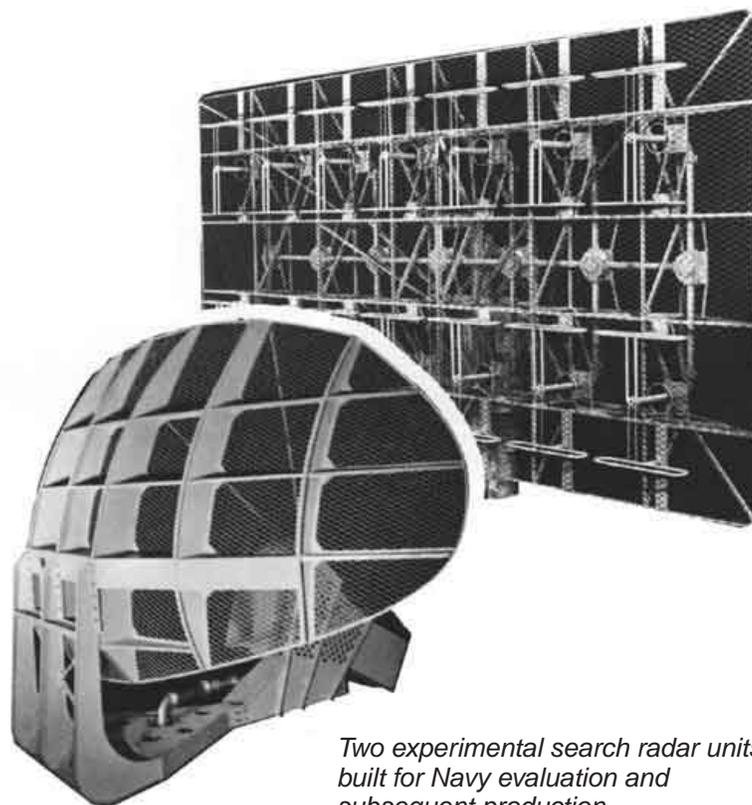
*Two experimental search radar units built for Navy evaluation and subsequent production*
