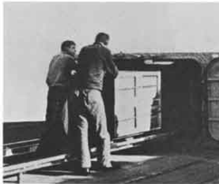
Pushline load enters elevator. Standard transfers and turntables permit varied layouts.
