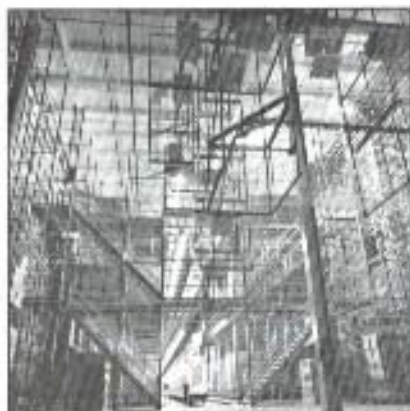
World's largest textile item order picking system combines Palletflo, Cartonflo and stackers in an integrated 3 floor level system. 1 million items in live storage permit rapid response to orders.
