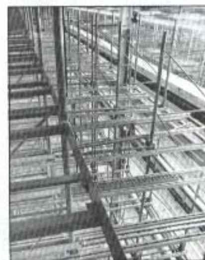
High cube live storage possibilities of Palletflo are dramatized in this installation photo.
