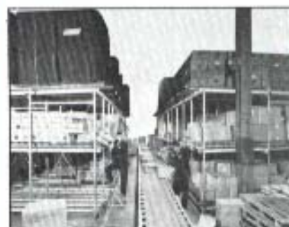
Two-level order picking from Palletflo for a restaurant chain. The third tier is last-in first out with access to the pallets of flat cartons from rear of rack.
