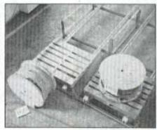
Pallet on Palletflo comes to a gentle stop. Uncontrolled load tumbled off pallet.
